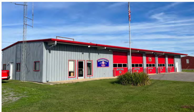
Typical of Essential Services areas.
